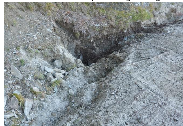
Photos 9 – Dish channel sump area filled in
