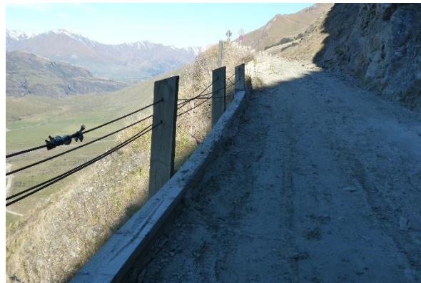
Photo 7 – Hardfill to deep next to guard log
