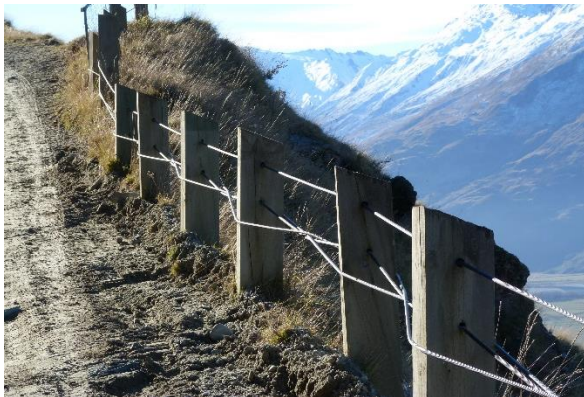
Photo 6 – Guard cables relatively tight
