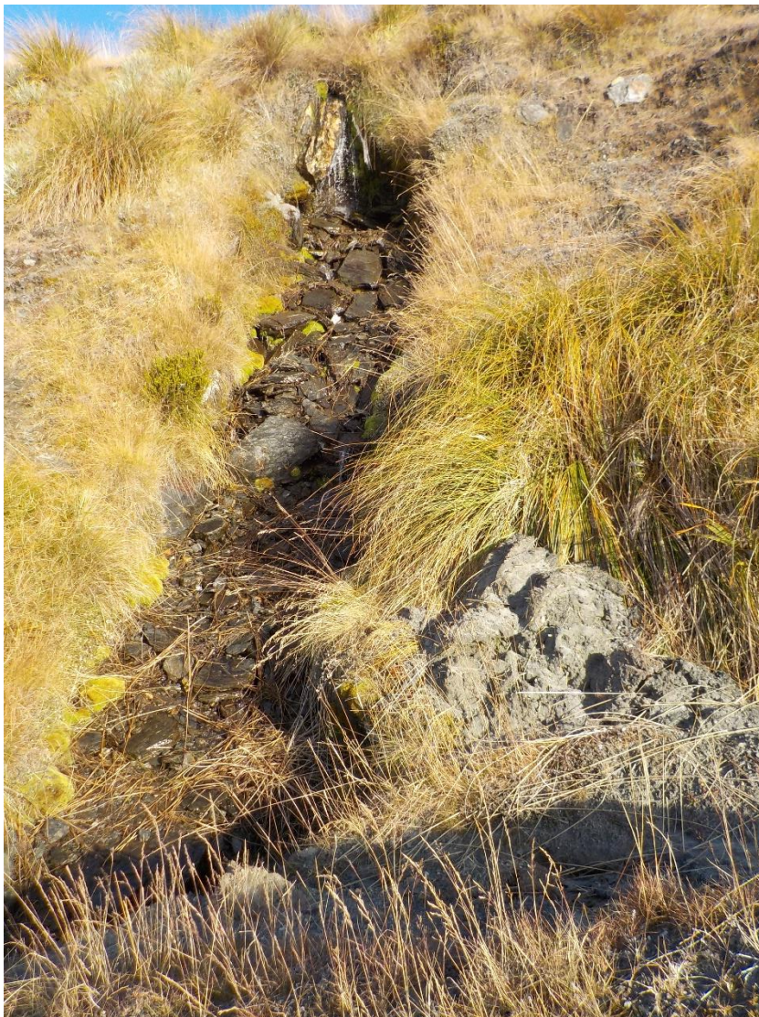
Figure 2: Site CONE1, a modified channel on the access track.
