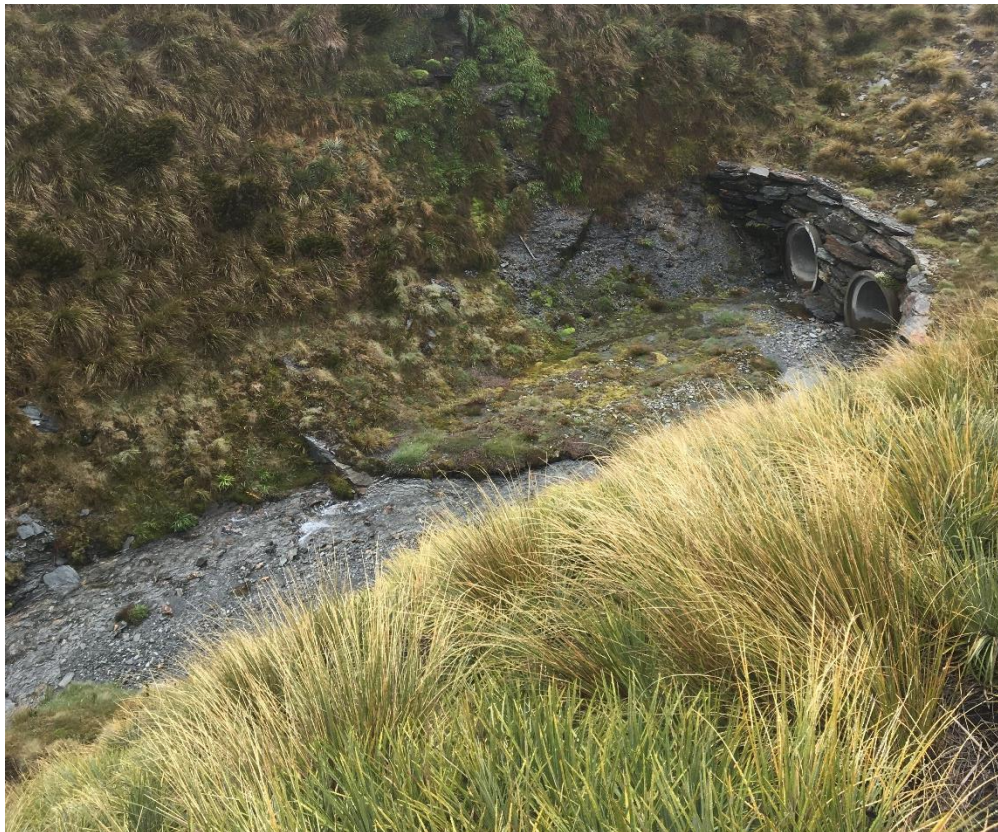
Figure 3: The clean stream bed upstream of the service track culvert.
