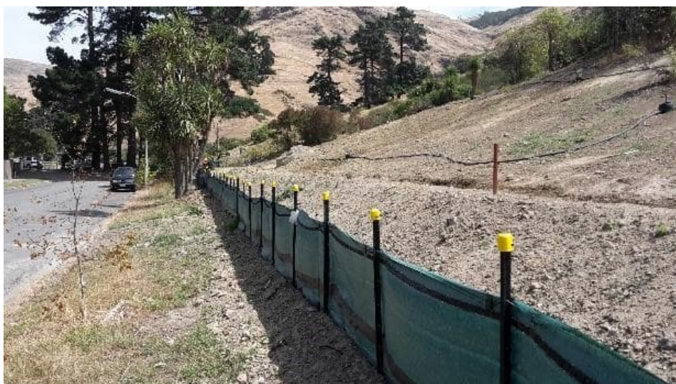
Figure 4-5 Silt fence example (Source: ECan ESC Toolbox)
