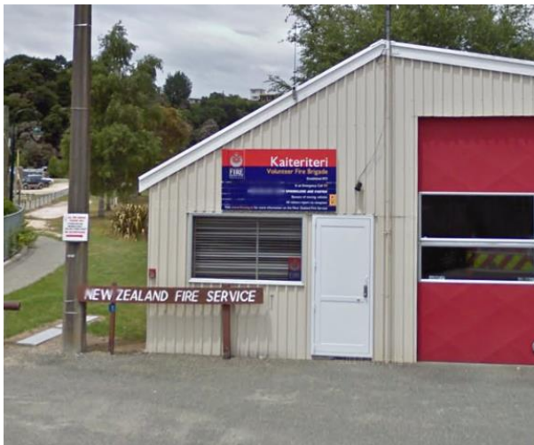
Kaiteriteri Volunteer Fire Brigade Building - Inlet Road, Kaiteriteri (Kaiteriteri Recreation Reserve)
