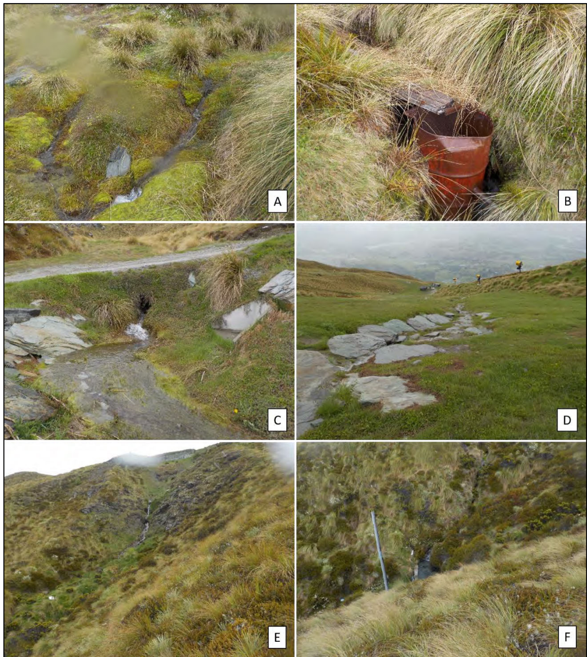
Plate 8: Stream 1. A – Springs at the stream source. B – Disused instream infrastructure. C – Track and culvert. D – Highly modified reach of Stream 1. E – Tributaries and waterfalls downstream of the access road. F – Water intake weir.
